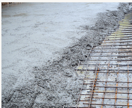
FIGURE 43 Detail image of ramp base construction
