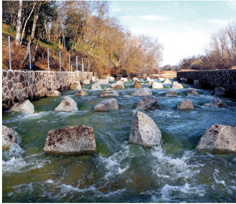
FIGURE 39. Ramp view, with the lateral walls covered with rocks
