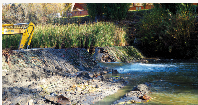
FIGURE 42 Partial demolition of the weir, aimed at pool emptying and cofferdam construction
