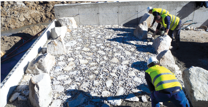
FIGURE 47 Covering ramp bed with rocks
