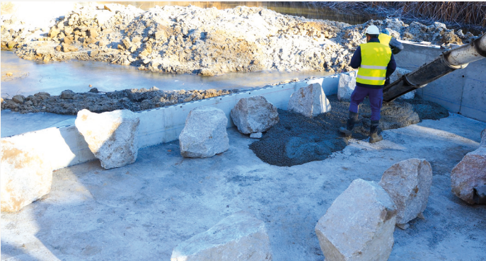
FIGURE 46 Ramp bed concreting
