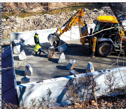
FIGURE 44 Placement of boulders in the ramp
