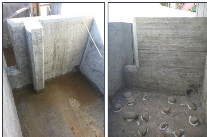
Figure 83. Unnaturalised bed (left) and bed naturalised by embedding stones (right).
