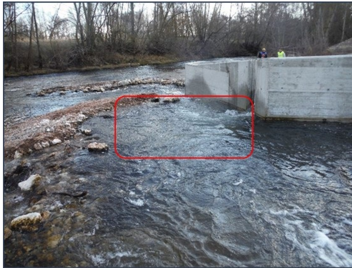
Figure 18. View of the pool in the river at the entrance (in red) of a fish pass.
