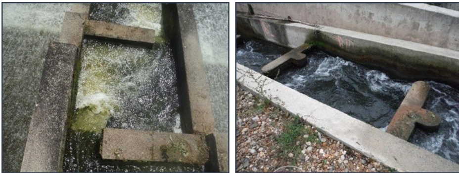
Figure 80. Pools with sharp edges (left) and rounded edges (right).
