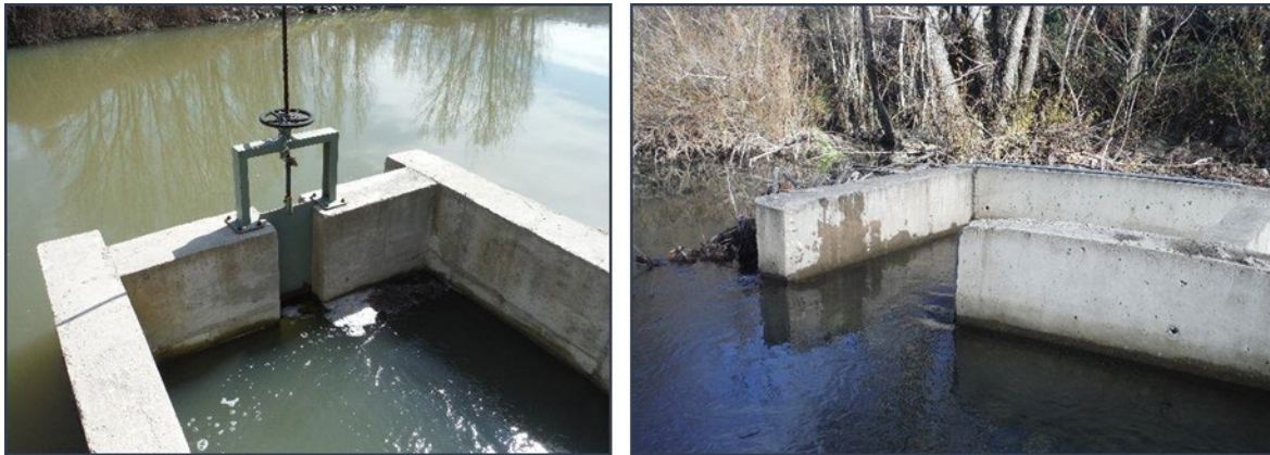
Figure 45. Fish pass exits with different widths: 20 cm (left) and 50 cm (right).
