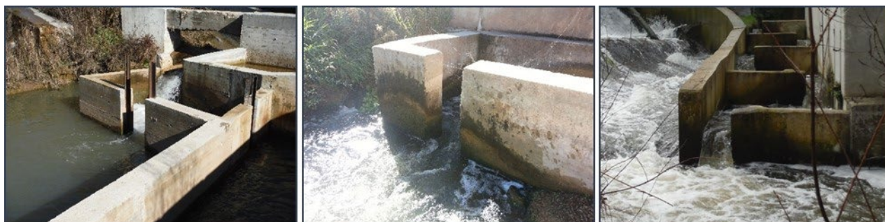
Figure 9. Difference in water level at the entrance: small (left); suitable (centre) and too large (right).
