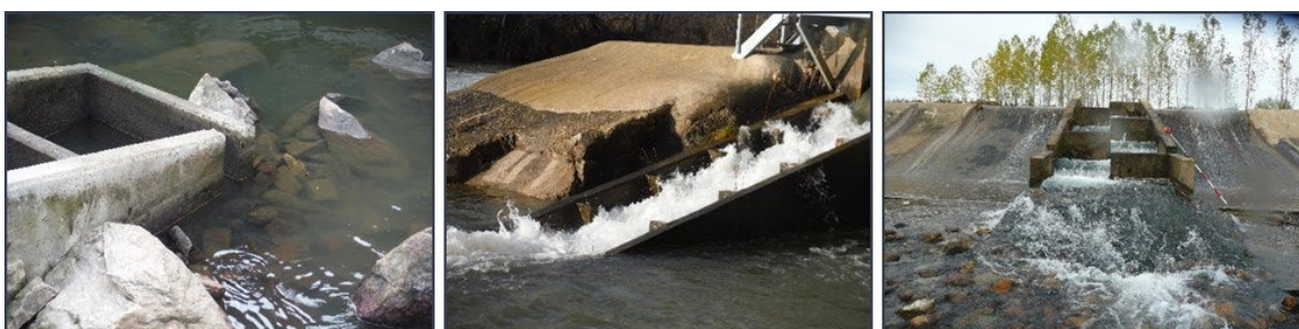
Figure 15. Entrances with different widths: 20 cm (left), 80 cm (centre) and more than 100 cm (right)
