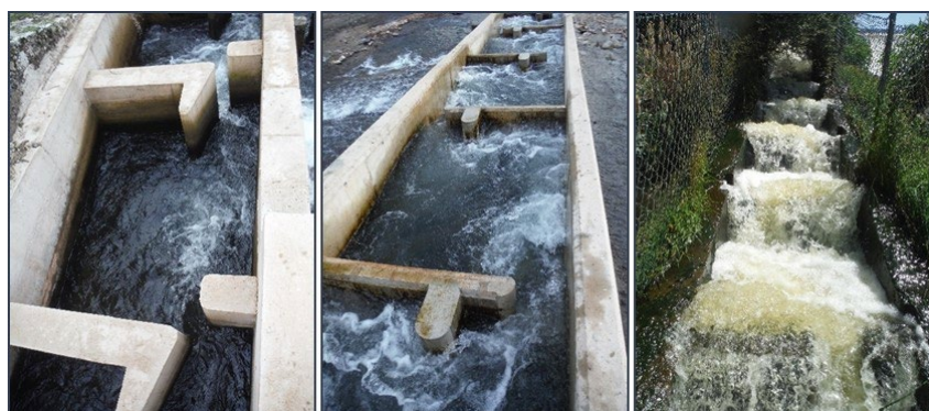
Figure 26. Pools where the volumetric power dissipation has a low value ( < 50 \text{ W}/\text{m}^3 ) (left), a typical value ( 150 - 175 \text{ W}/\text{m}^3 ) (centre) and a too high value ( > 350 \text{ W}/\text{m}^3 ) (right).
