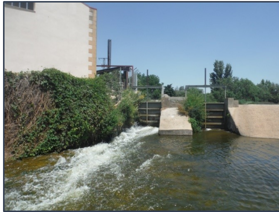
Figure 56. Gates to empty the weir, located on the bank opposite from the fish pass, next to the hydropower station.
