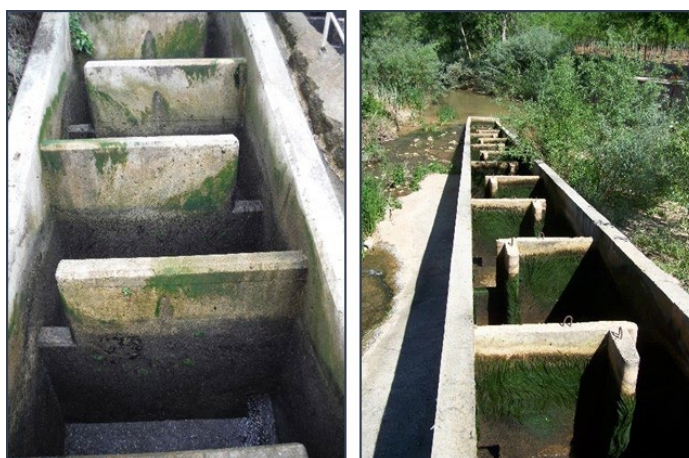
Figure 82. Pools without baffles (left) and with them (right).
