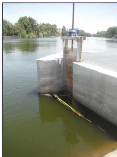
Figure 58. Gate and baffle at the point where fish exit, that is, where water goes into the fishway.
