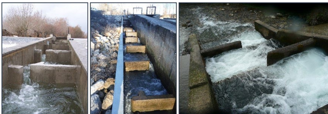
Figure 34. Openings connecting pools with different widths: 20 cm slots (left), submerged notches, also 20 cm wide (centre), and surface notches, 133 cm wide (right).
