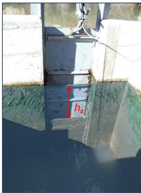
Figure 42. Depth at exit seen from the inside of the fish pass (closed gate).
