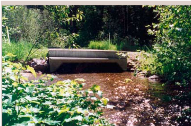
Figure 4.8—Brewster Creek road replacement box culvert, filled to 85 percent of its rise after 1 year.
